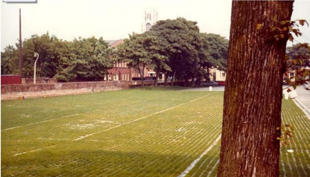
Figure1. Installed grasscrete paver.
